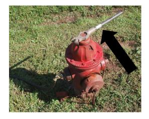
a tool the firefighters use to get water from a hydrant
